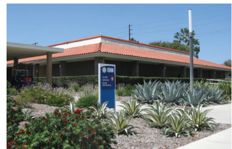
The MWDOC Administration Office is an existing 3,000 sf area that will be modernized to improve operational efficiencies, office workflow, and meet the agency’s needs of current and future staff.
