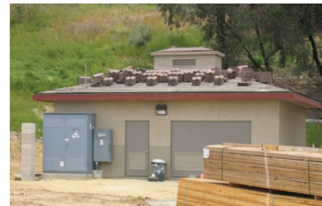
City of Orange Carver Pump Station during construction
