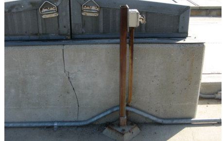
Inland Empire Utility Agency, RP-1 Primary Clarifier
